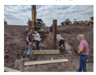
Once the support is built, the pipe is then laid and tamped.
