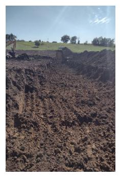
With larger dams, a sand drain and collar are installed for the pipe. A collar is a fifteen-foothigh sand wall that stops and outlets the water from the pond into the drain. The picture below shows the collar being dug.
