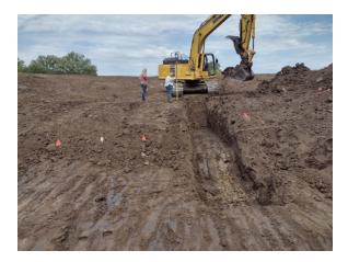
The end of the drain has a small gravel filled area with riprap on the end.
