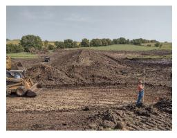
Next, the dam is finished, a trash rack is placed over the pipe, and the land surrounded the pipe is seeded. With this step, mulching is highly recommended.
