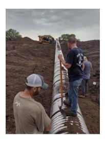
After the pipe is laid, the pipe support is finished, and then the workers begin bringing in fill and building up the sand collar, four feet at a time. This requires putting in fill dirt, then digging back down to the collar, and continuing to place the sand. When doing this, it is always a good idea to mound up some waste sand over the pipe before digging down the first time, so that the backhoe does not damage the pipe.
